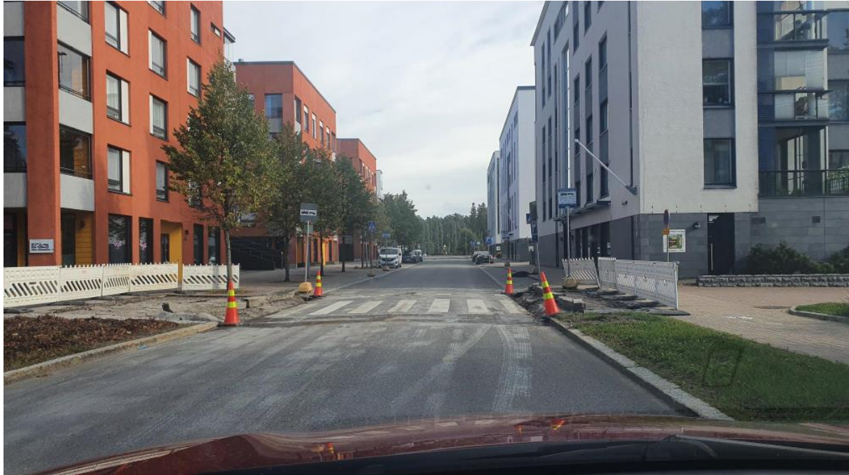
Figure 13: Roadwork on the robobus's route
